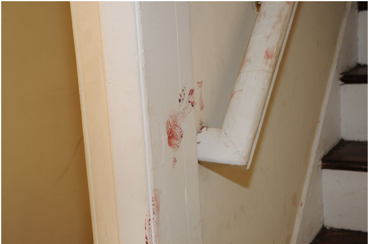
Staircase Leading to Third Floor
