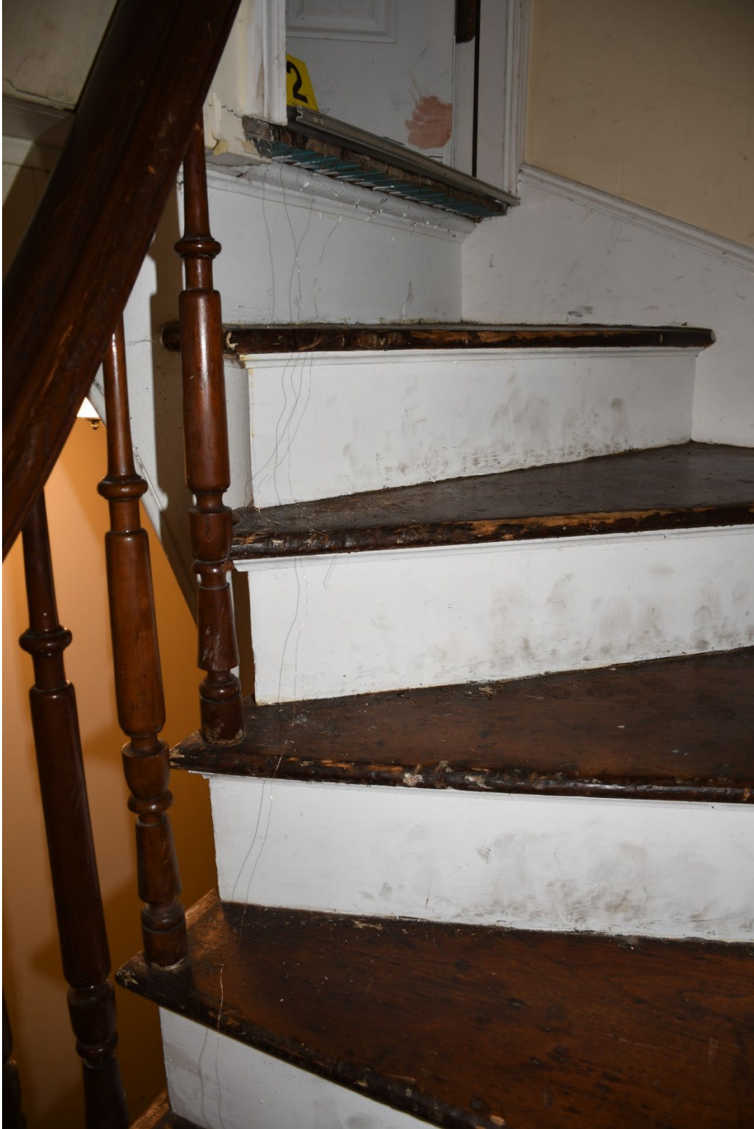
Second Floor Landing
