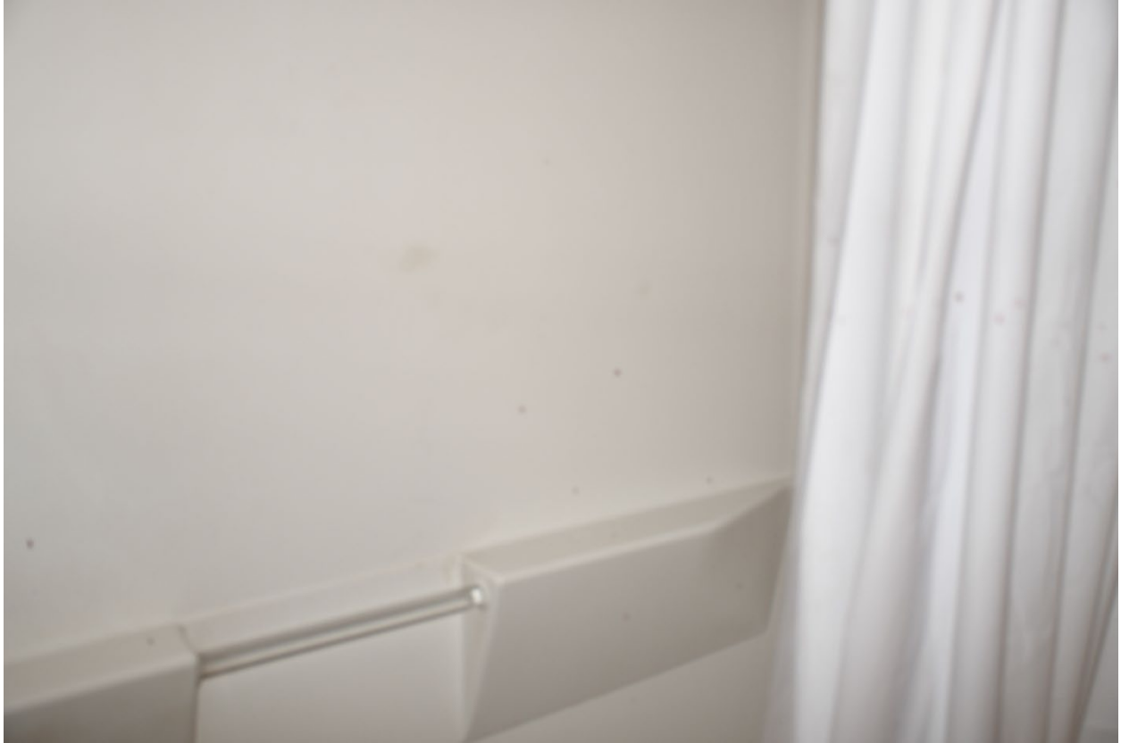
Third Floor Tub/Shower
