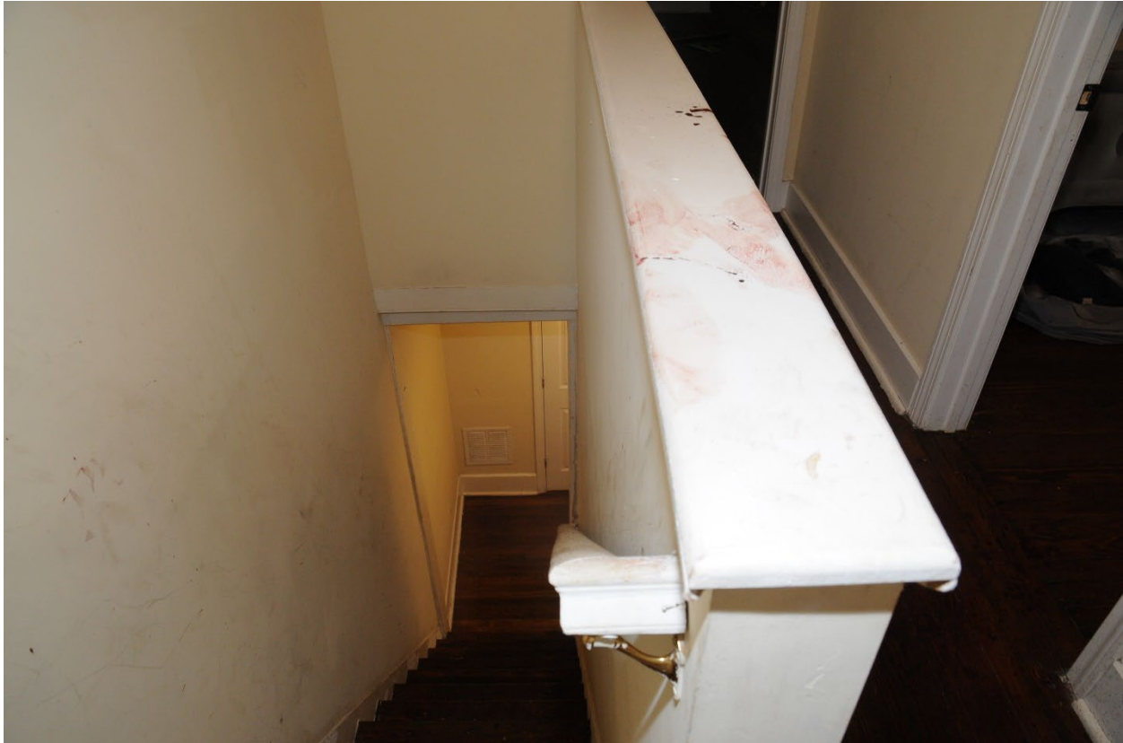
Half Wall on Third Floor
