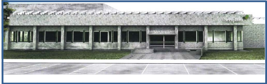
Planned Theraplant building, Watertown
