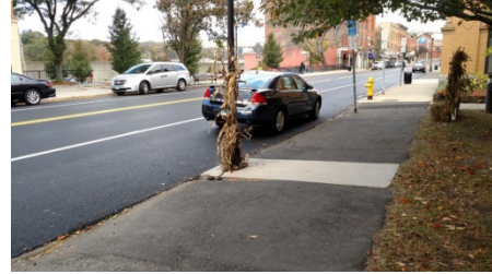
Figure 16. Curbcut in Front of Senior Center
