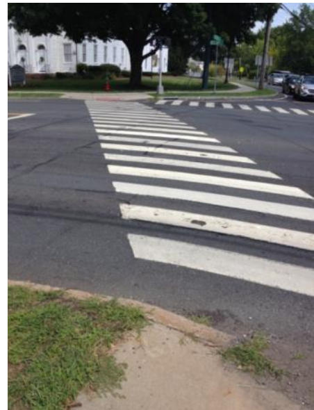
Figure 31. Crosswalk on Rt. 44 west of
