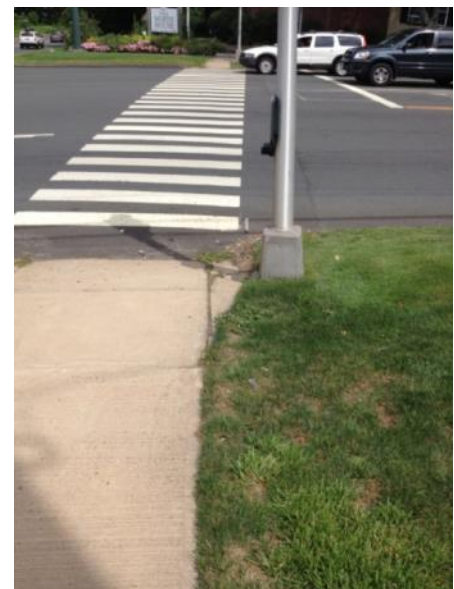
Figure 37. Crosswalk between Avon Old Farms Hotel (near side) and North House (far side) across Rt. 44 east of Old Farms Road
