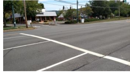
Figure 36. Intersection of Route 44 and Fairway Shops
