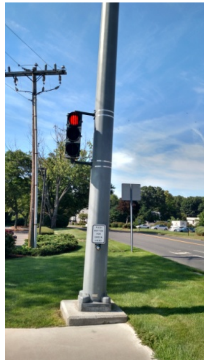
Figure 20. Pedestrian pushbutton on the east leg of West Main Street
