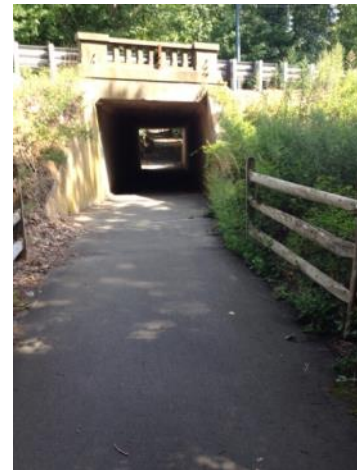
Figure 27. Multi-use path looking north under Route 44 west of Darling Drive
