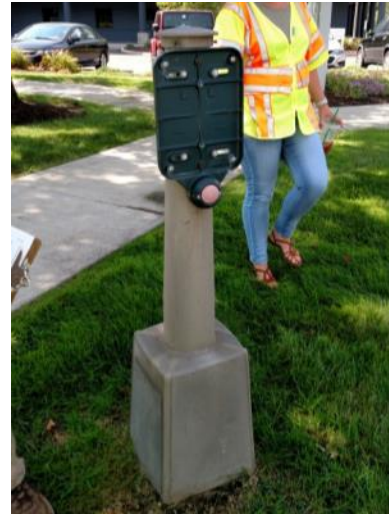
Figure 21. Inadequate pedestrian pushbutton in the south east corner at Fox Hollow
