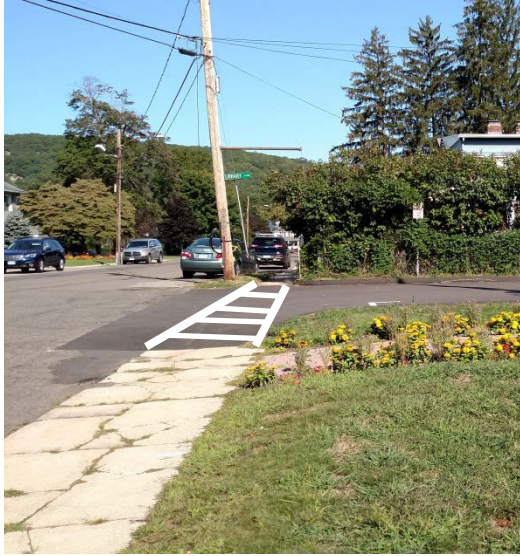
Figure 13. Paint a Crosswalk
