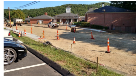
Figure 6. Highland Avenue Reconstruction
