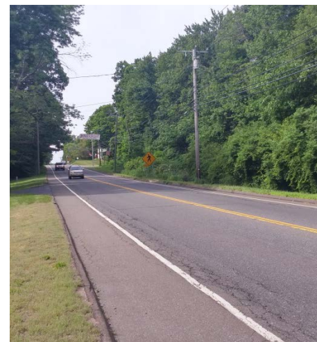
Figure 9. Good Sightlines for Northbound Traffic at Library
