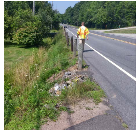
Figure 10. Open Drainage Ditch on Bolton Center Road
