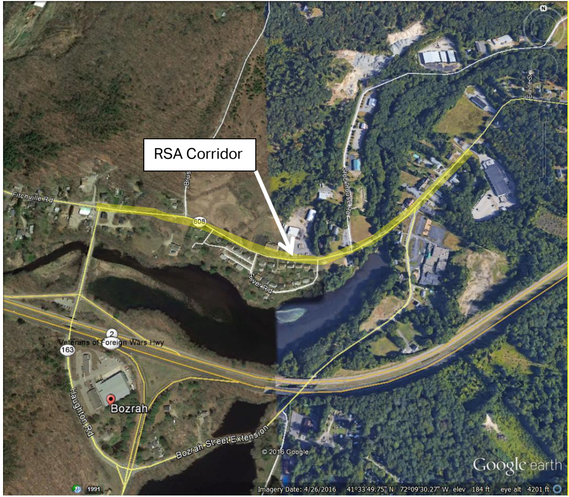
Figure 1. Fitchville Road (State Route 608), Bozrah
