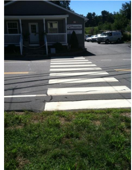
Figure 11. Mid-Block Crosswalk east of Bozrah Street Extension
