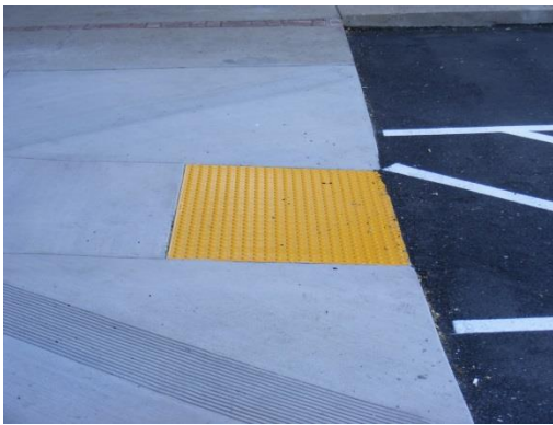
Figure 16. Tactile Warning Strip
