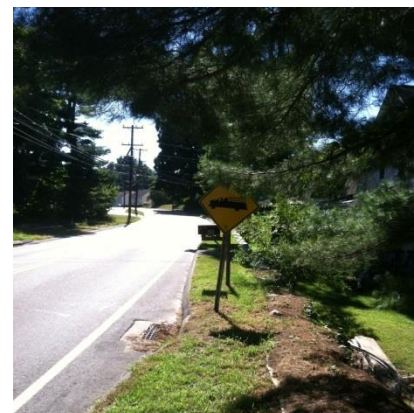
Figure 8. Older Signs Lacking Retro-Reflectivity
