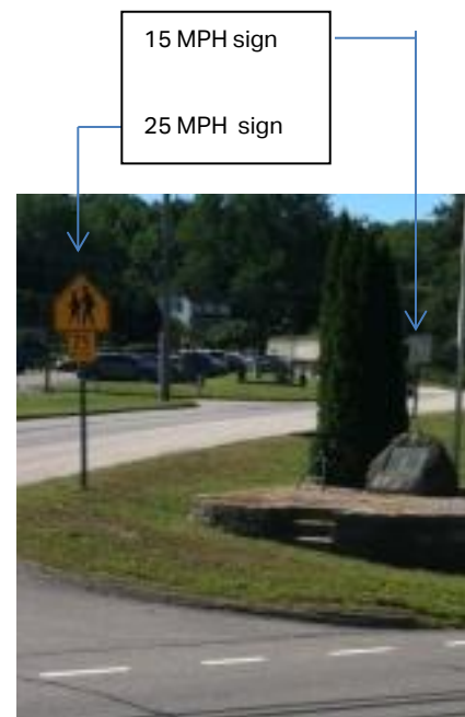
Figure 5. Conflicting Speed Limit Signage
