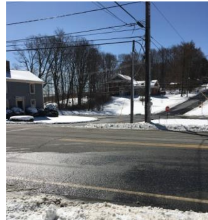
Figure 6. Visibility reduced by location of utility poles
