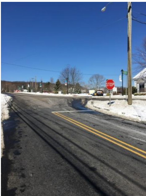
Figure 17. Add bump-out on southwest corner and pavement markings at George Washington Turnpike/Route 4
