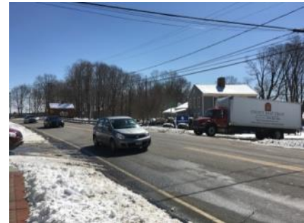
Figure 10. Narrow shoulders on Route 4
