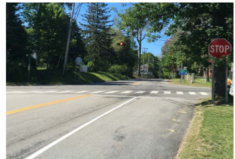
Figure 8. Example of Wide Shoulder Southbound on Route 169 Used as Right-turn Lane at the Intersection
