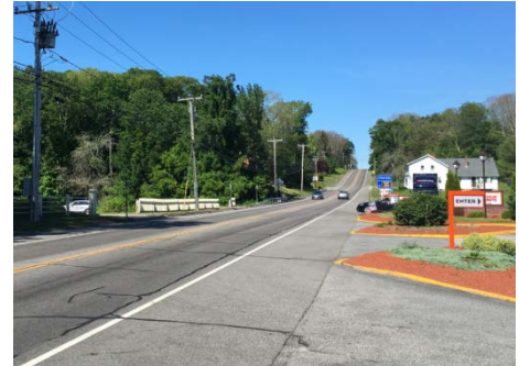
Figure 6. Multiple Driveways Facing West on Route 14.
