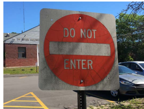
Figure 11. Faded Sign Wear at Middle School Exit Driveway
