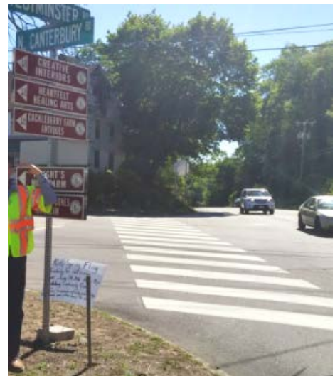
Figure 7. Existing Crosswalk Without Ramp on Route 169
