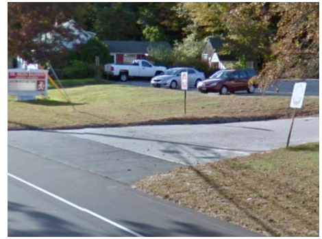
Figure 9. “Do Not Enter” Signs Set Too Far Back at Middle School Exit Driveway
