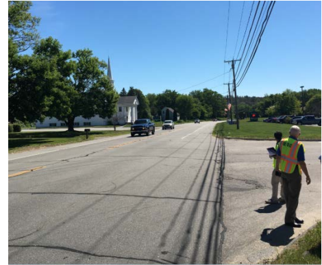
Figure 13. Lack of Sidewalks on Route 14 at Canterbury Plains Shopping Center
