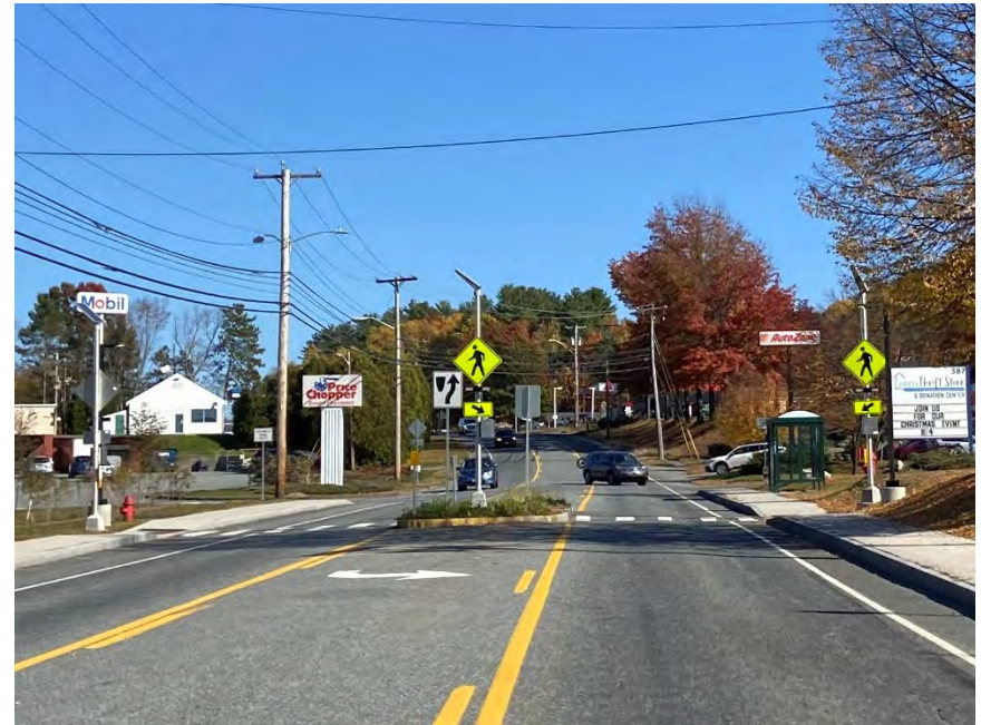
Exhibit 45: A pedestrian refuge island on US Route 4 in Lebanon, NH
