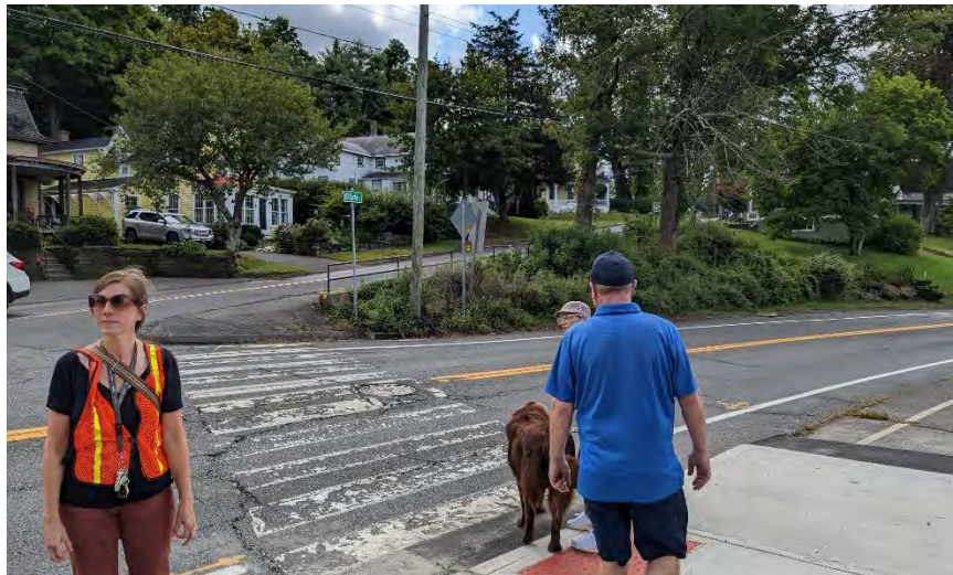
Exhibit 19: New curb ramps at Route 179 (Bridge Street) at Center Street
