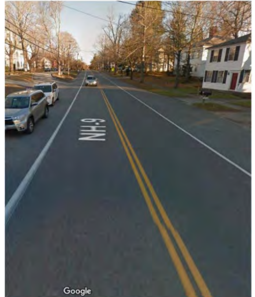
A 10-ft lane installed in Hopkinton, NH
