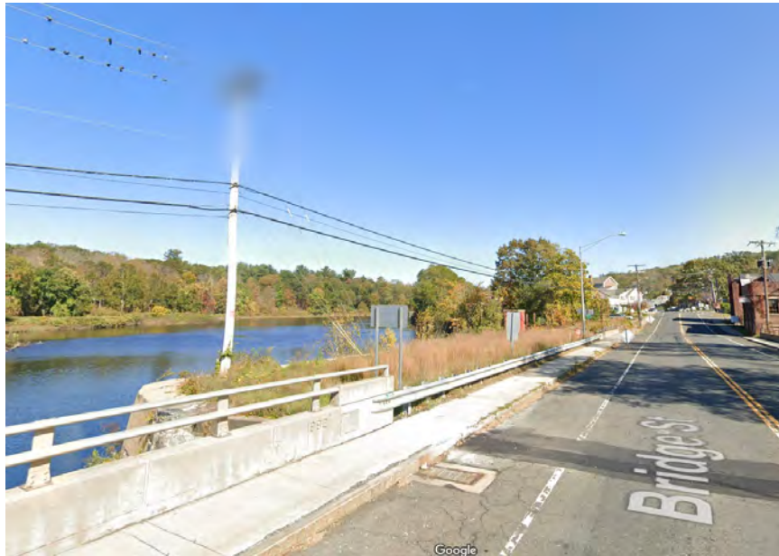
Exhibit 32: Consider this location for a pocket park between these two bridges. Locate gateway signage in this location to give visual cues to motorists entering Downtown from this direction. Source: Google Maps Streetview
