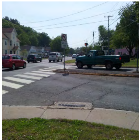
Exhibit 5: A photo from the 2016 RSA showing the pedestrian crossing of River and Bridge Streets.
