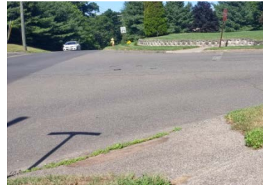
Figure 13. Guinevere Ridge Pedestrian Crossing
