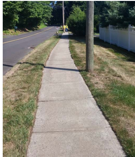
Figure 11. Jarvis Street existing sidewalk
