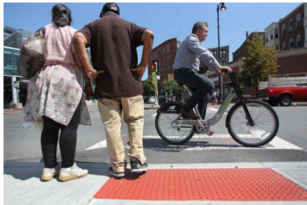
Figure 16. Pedestrian Detectable Warning Strips
