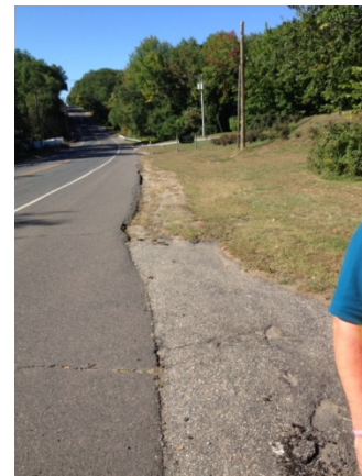
Figure 12. Route 66 Looking East Towards Senior Center
