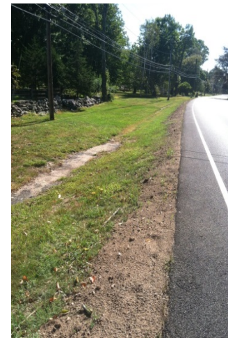
Figure 18. Existing Swale on East Side of Route 87 Near #255.
