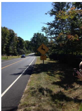
Figure 19. Low Mounted Sign on Route 87
