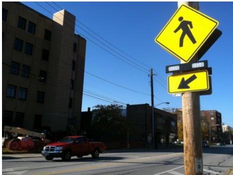
Figure 15. Rectangular Rapid Flashing Beacon
