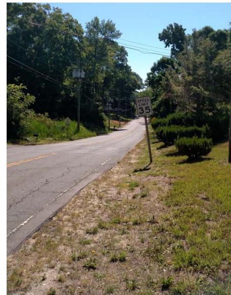
Figure 8. South Side of Route 31
