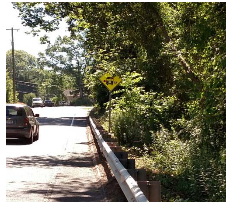
Figure 7. Sign Blocked by Vegetation
