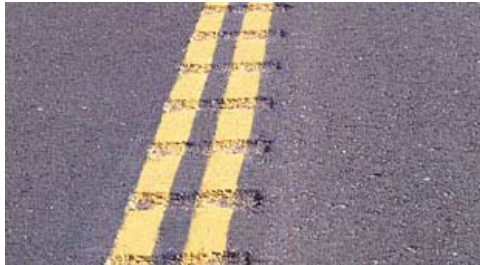
Figure 23. Example of Center Line Rumble Strips
