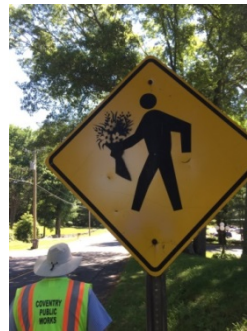
Figure 18. Replace Sign with Retroreflective Ones
