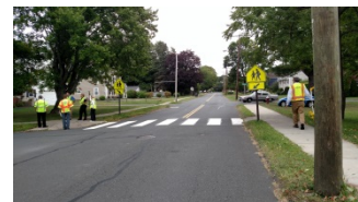
Figure 7. Crosswalk connecting sidewalks at Raymond Place
