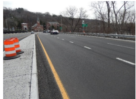
Figure 26: Route 34 eastbound over Atwater Bridge
