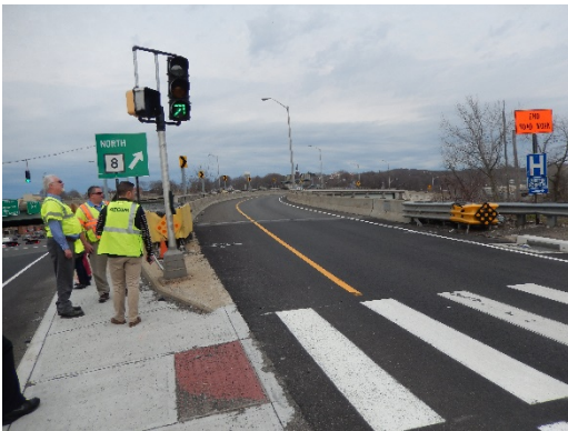
Figure 25: Pedestrian accommodations on Route 8 On-Ramp
