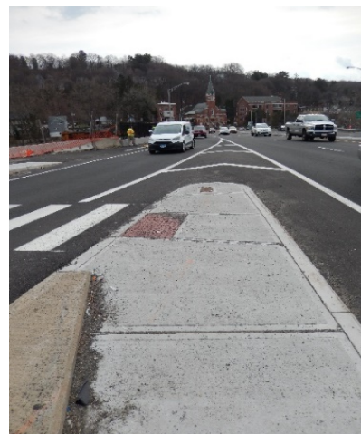
Figure 16: View of westbound traffic on bridge and entering Route 8
