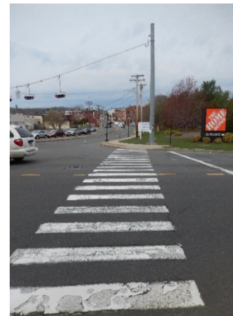
Figure 12: Crosswalk at Home Depot Entrance
