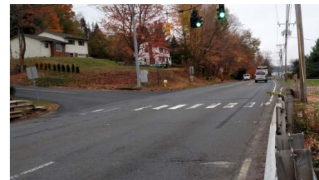
Figure 12. Mountain Road Intersection
