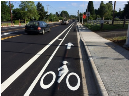
Figure 25. Painted Buffer Between Travel Lane and Bike Lane
