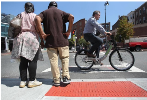
Figure 27. Ramp and Detectable Warning Strip
