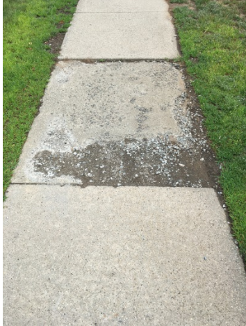
Figure 17. Repair Damaged Sidewalks
