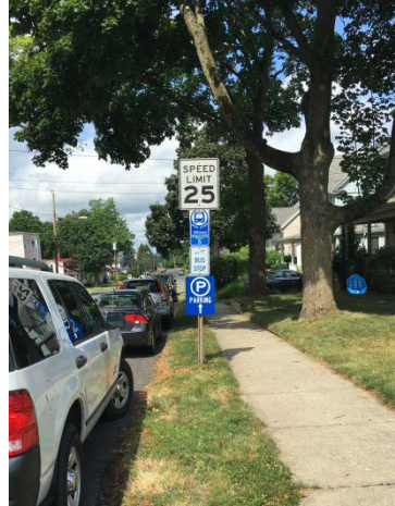
Figure 18. Raise Signs to Standard Height
