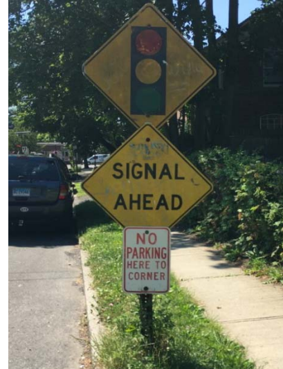
Figure 15. Signs mounted below standard height
