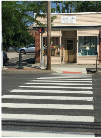
Figure 6. Crosswalk and detectable warning strips
