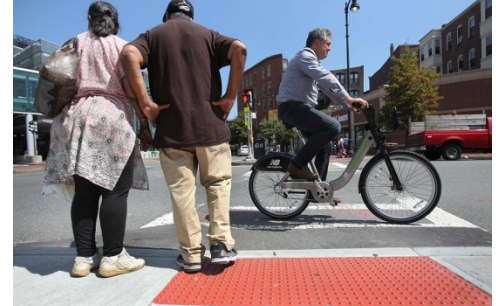
Figure 21. Typical detectable warning strip
