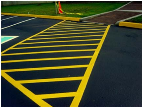
Figure 18. Paint no parking pavement markings
