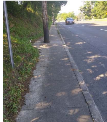
Figure 8. Narrow sidewalks/utility poles in
