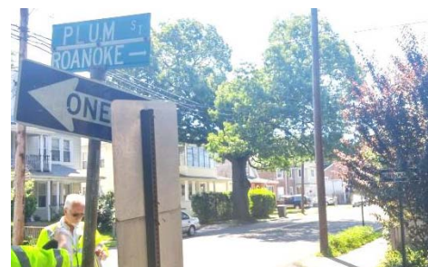
Figure 14. One Way Sign pointing in wrong direction/covered by branches
