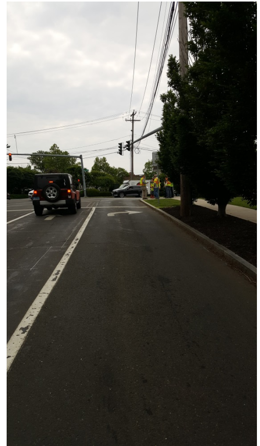
Figure 9 Overgrown Vegetation Blocking Signs
