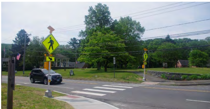
Exhibit 18: Route 154 crosswalk with an RRFB south of former Elementary School entrance
