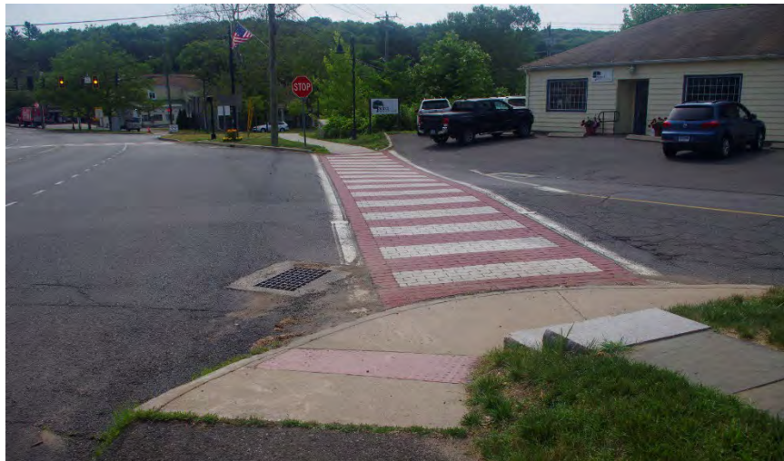
Exhibit 21: Crosswalk at the intersection of Route 154 and Candlewood Hill Road
