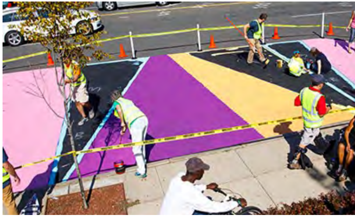
Exhibit 33: An example of a painted bump out used to slow traffic and shorten crossing distances for pedestrians in Hartford (Source: FHI Studio)
