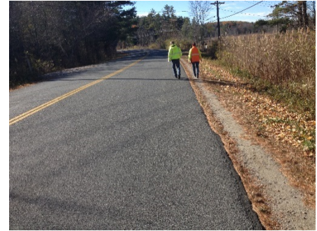
Figure 5: Looking north on White's Woods Road toward Greenway crossing
