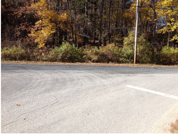
Figure 12: Webster Road approach to White's Woods Road
