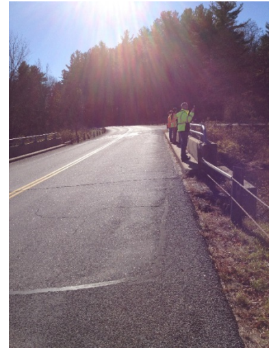
Figure 10: Bridge on White's Woods Road looking south
