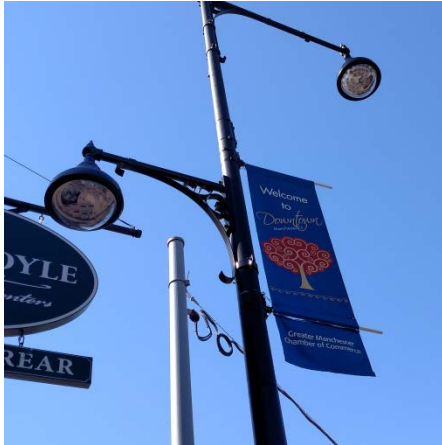
Figure 7. New LED Lighting Being Installed
