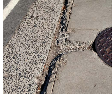
Figure 9. Deteriorating Curbing
