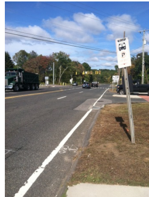
Figure 9. Bus stop sign in poor condition
