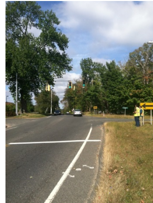
Figure 13. Signs lacking retro-reflectivity
