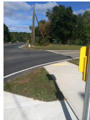
Figure 19. No receiving ramp on Route 320 north side
