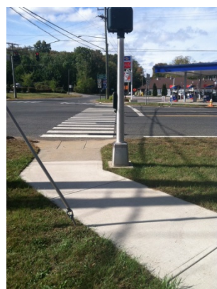
Figure 7. Long crosswalk, no detectable warning strips
