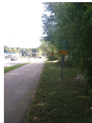
Figure 17. Multi-use path signs obstructed by branches
