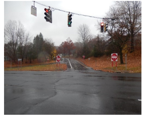
Figure 12: I-84 eastbound off-ramp
