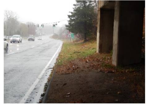
Figure 11: I-84 abutments on west side of Route 63
