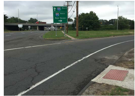
Figure 12. I-95 Ramp Crossing
