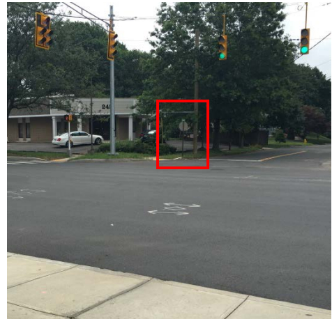
Figure 15. Stop Sign not Removed When Signal Installed at Corona Drive
