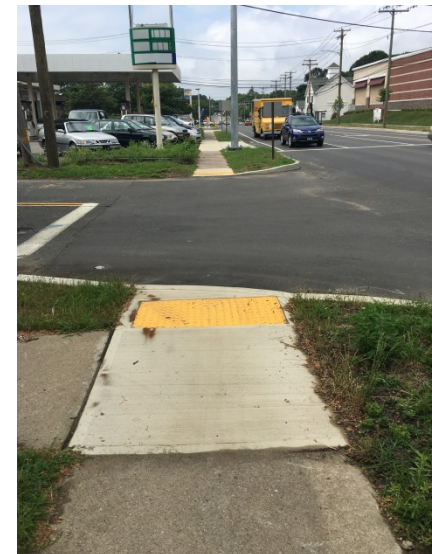
Figure 14. No Pedestrian Crosswalk and Signal at Corona Drive
