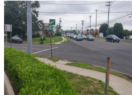
Figure 7. No Crosswalk and Non ADA Compliant
