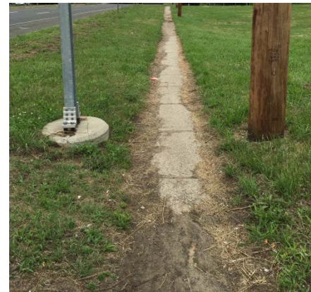
Figure 13. Sidewalk Between I-95 Ramps
