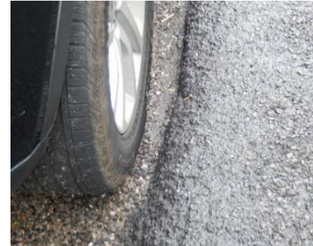
Figure 9. Drop from road edge to gravel parking lot
