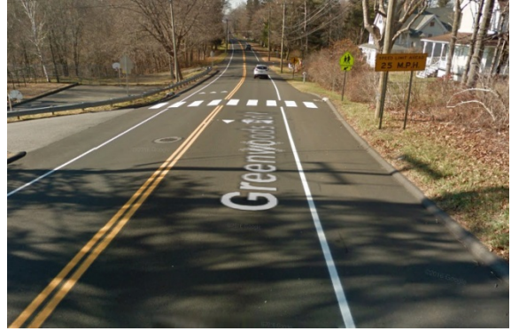
Figure 5: Greenwood Road East looking westbound in front of Botelle Elementary School
