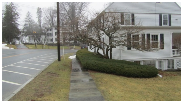
Figure 17: Greenwood Road east looking west at shrubs growing over slate sidewalk at #3 and diagonal striping to designate no parking
