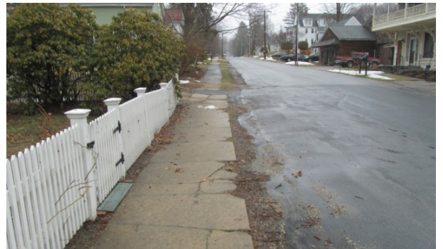
Figure 14: Sidewalk on the west side of Maple Avenue
