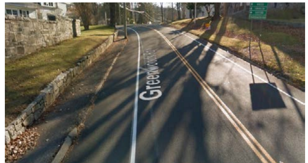
Figure 19: Greenwood Road West looking south with sidewalk and retaining wall on the left (east) side
