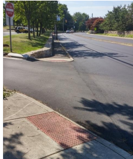
Figure 7. Curb Ramps at Elementary School Exit Driveway
