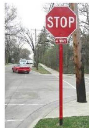
Figure 11. Example 4-Way Stop Sign With Reflective Post
