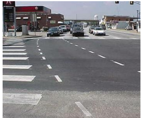
Figure 13. Example "Cat track" Lane Markings
