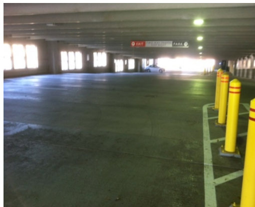
Figure 13. Transportation Center parking garage
