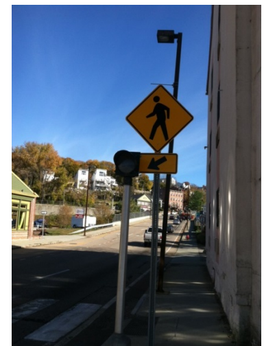
Figure 12. Constant flashing beacon at mid-block crosswalk
