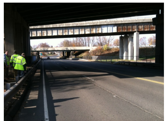
Figure 18. I-84 overpass of Route 536
