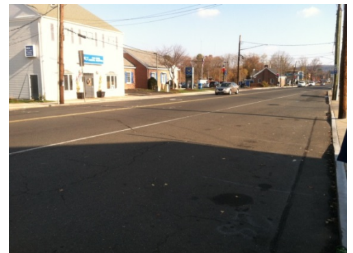
Figure 6. Route 372 looking east
