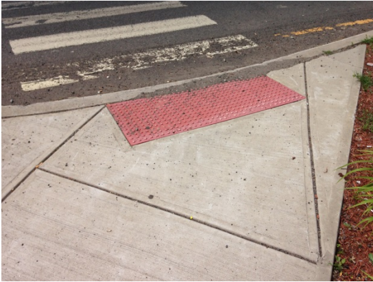
Figure 20. Tactile warning strip
