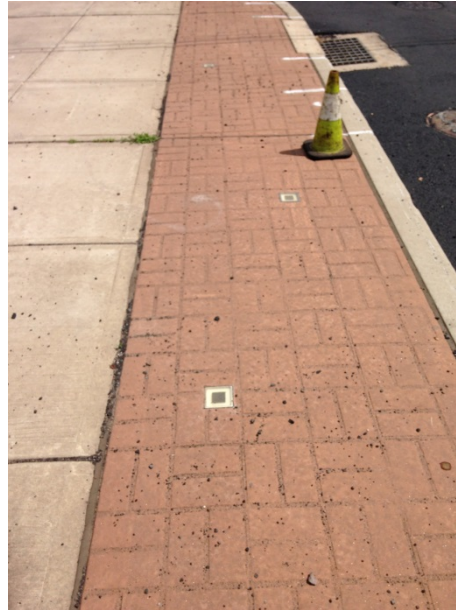
Figure 6. Lights installed in sidewalk
