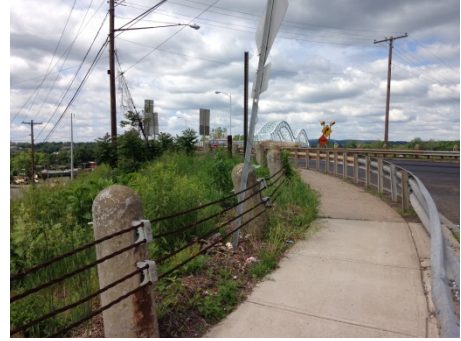
Figure 10. View of approaching vehicles at the Arrigoni Bridge and Lower Main Street crosswalk
