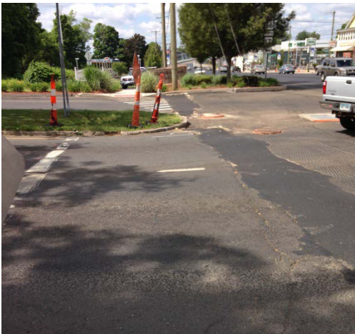
Figure 22. Crossing on Marlborough Road at Main Street intersection
