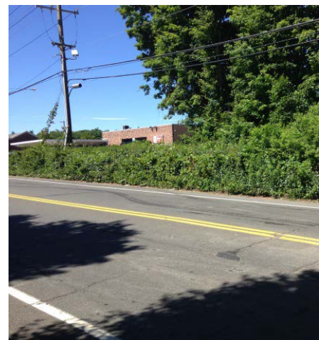
Figure 7. Overgrown Stone Wall
