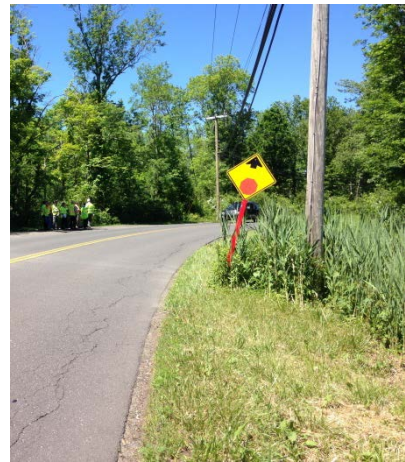
Figure 9. Existing Advanced Intersection Warning
