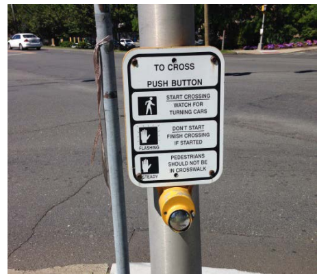
Figure 11. No ADA Compliant Button
