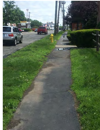
Figure 14. Pooling on Sidewalk
