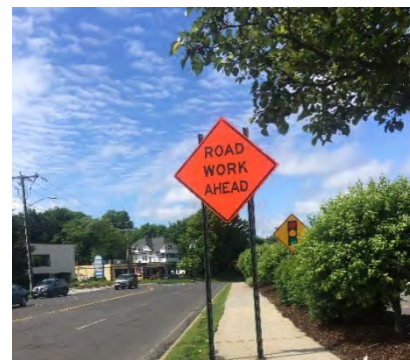
Figure 11. Sign Blocked by Vegetation
