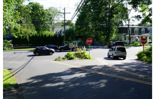
Figure 2-7 Small pedestrian refuge island
