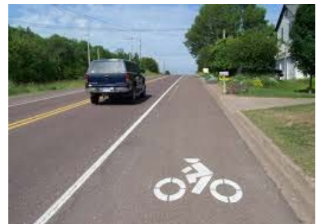
Figure 11. Typical Bicycle Lane
