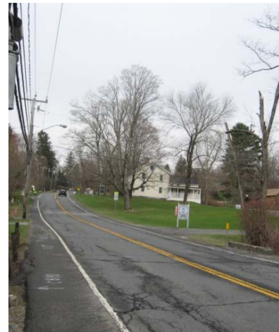
Figure 5. Deteriorating Pavement
