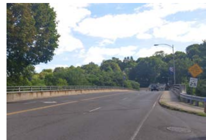
Figure 11 - Broad Street Bridge
