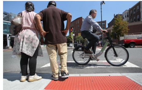
Figure 20 - Tactile Warning Strip
