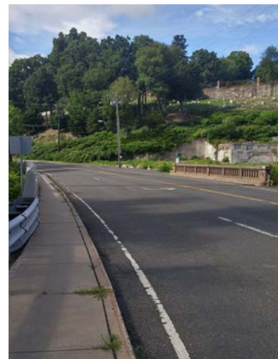
Figure 7 - River Street Bridge
