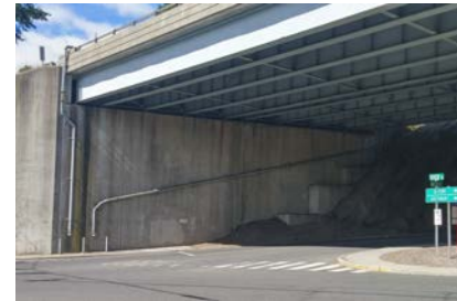
Figure 10 - West Street Approach
