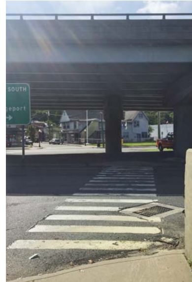
Figure 6 - Wakeley Street under
