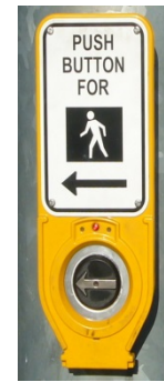
Figure 19 - Pedestrian Signal Equipment
