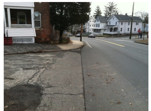
Figure 25: Tree restricting sight distance
