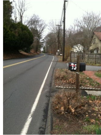
Figure 6: Utility poles close to road
