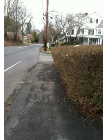
Figure 14: Hedge encroaching over sidewalk at 79 Shelton Avenue
