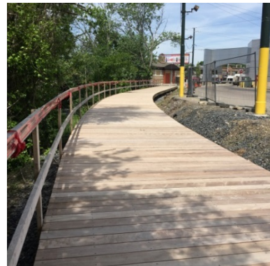
Figure 21: Example of cantilevered boardwalk above a river
