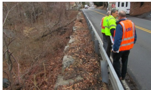
Figure 12: Rock structure directly behind the guiderail on the north side
