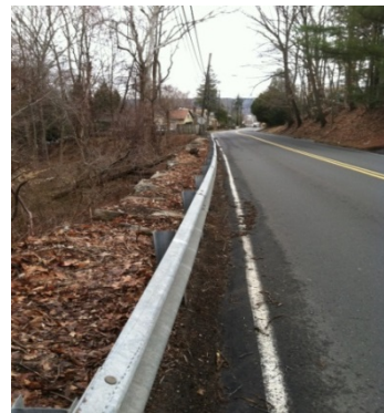
Figure 20: Stone wall behind guiderail
