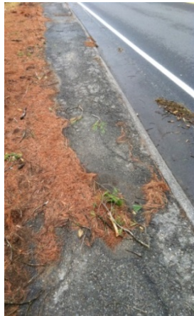
Figure 11: Existing bituminous sidewalk on Shelton Road near Meadow Street
