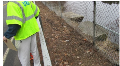
Figure 7: Grass area between the chain link fence and guard rail
