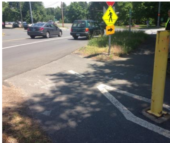
Figure 25. Add Wood Guardrail and Remove Bollard
