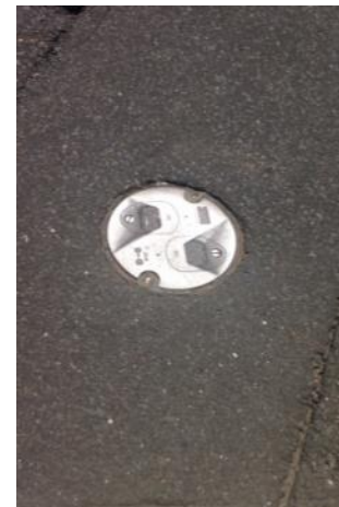
Figure 26. Replace LED Lights
