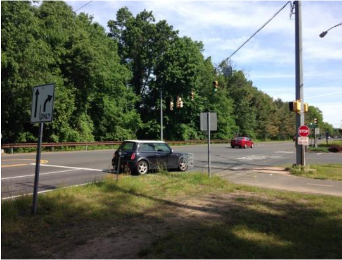
Figure 31. Tighten Turning Radius
