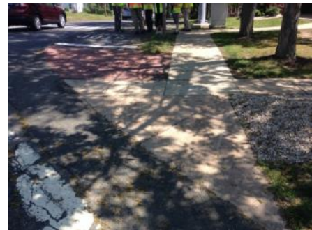
Figure 16. Sidewalk and Trail Have Multiple Surface Types
