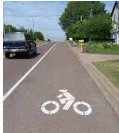
Figure 23. Paint Bike Symbols on Iron Horse Boulevard
