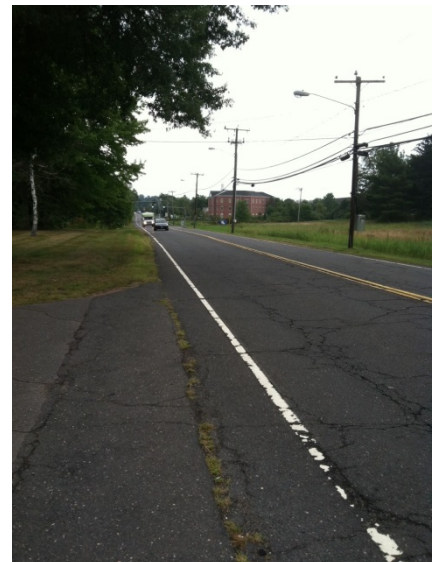
Figure 6. Ellington Road Facing East
