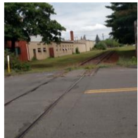
Figure 18. Rail Road Tracks Across Aircraft Road
