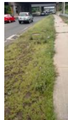
Figure 10. Grass Buffer/snow Shelf on West Side of Queen Street North of I-84
