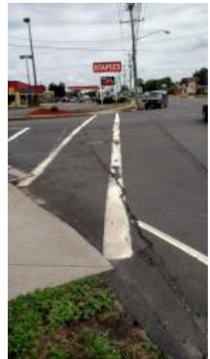
Figure 13. Crosswalk Across Spring Street at Queen Street
