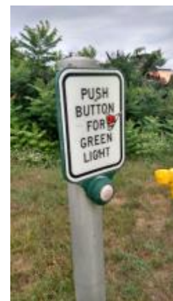
Figure 11. Pedestal With Pedestrian Push Button at Queen Street/I-84 Westbound Ramps (north)
