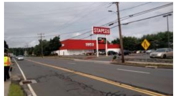
Figure 16. Spring Street Showing Lane Drop From Two to One Lane westbound.
