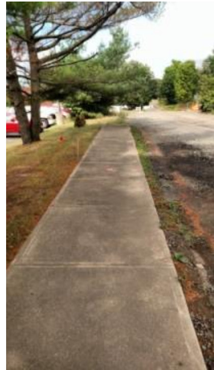
Figure 5. John Weichsel Crossing Looking West Showing Sidewalk and Road Construction
