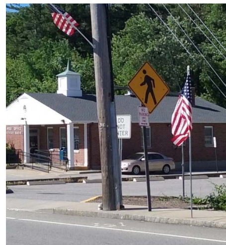
Figure 5. Utility Pole in Sidewalk Creating Pinch Point
