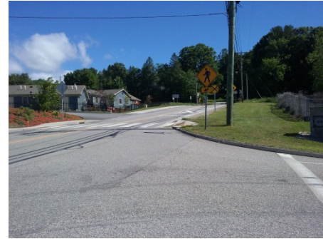
Figure 7. Crosswalk with no Sidewalk Connection to the Firehouse
