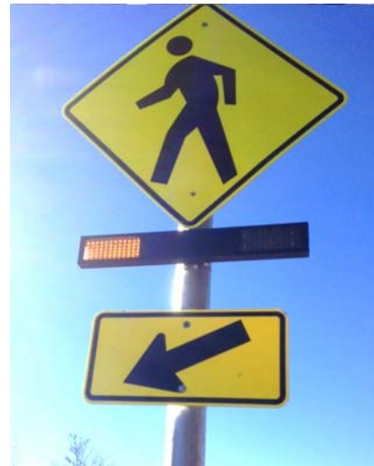
Figure 22. Active Pedestrian Crossing Sign
