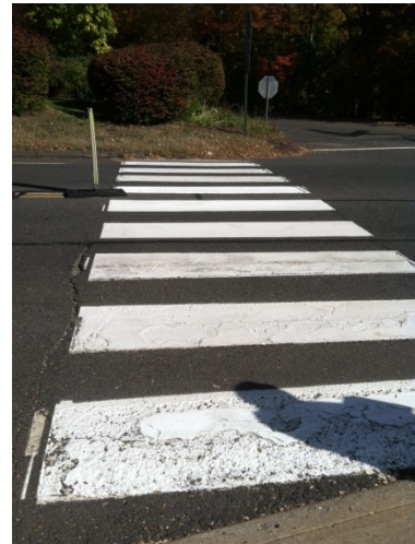
Figure 16. Crosswalk without ramp or warning strip
