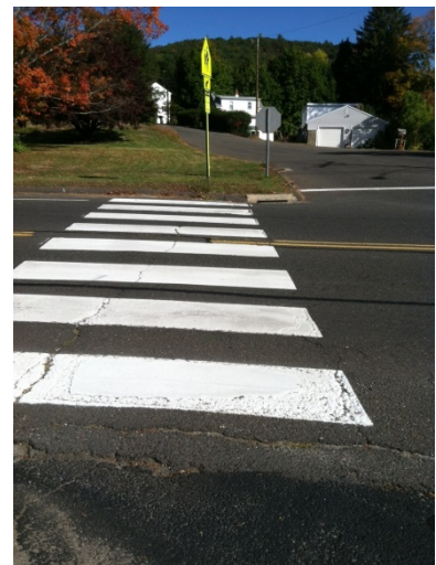
Figure 9. Crosswalk without ramp or landing
