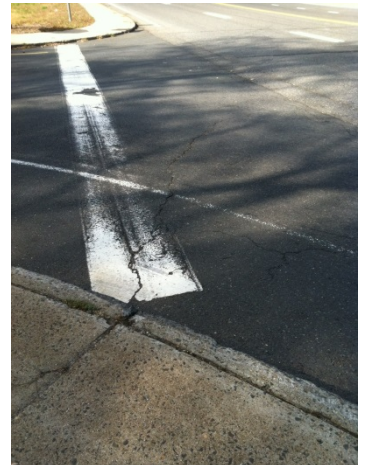
Figure 20. Sidewalks without crosswalk or ramps
