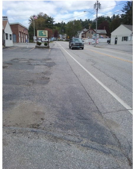
Figure 14. Large Curb Cuts at Cumberland Farms
