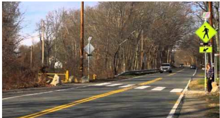
Figure 24. Active Pedestrian Rail Trail Crossing
