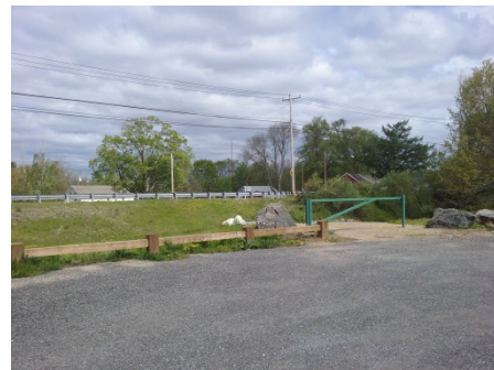
Figure 7. Lack of Lighting in Rail Trail Parking Area
