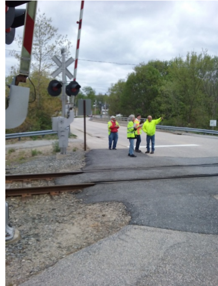
Figure 19. Stop Bar Set Back Behind Tracks
