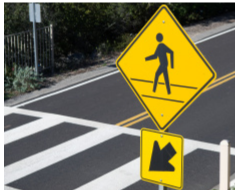
Figure 26. Pedestrian Crossing with Down Arrow Plaque
