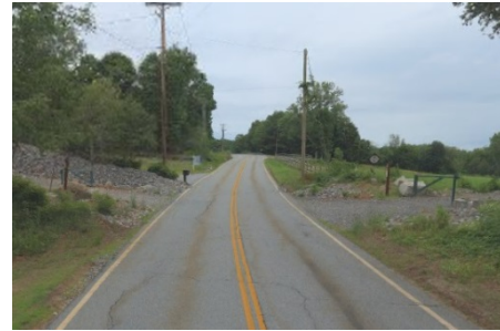
Figure 8. Airline Trail Crossing Route 193
