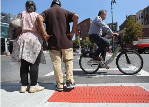
Figure 21. Example of Detectable Warning Strips
