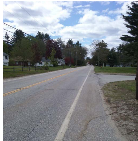
Figure 10. Lack of Sidewalks Along the Route 12 Corridor
