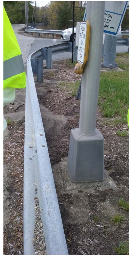
Figure 9. Crossing Push Button Behind Guide Rail
