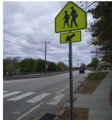
Figure 20. Non-ADA Compliant Ramp on Route 12 at Main Street
