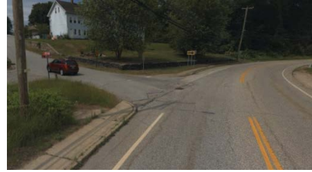
Figure 13. Intersection of Thatcher Road and Route 12
