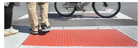
Figure 28. Tactile Warning Strip
