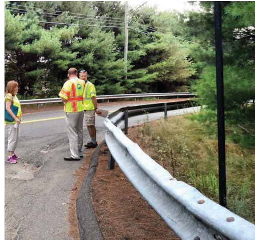
Figure 19. Fix Broken Guard Rail
