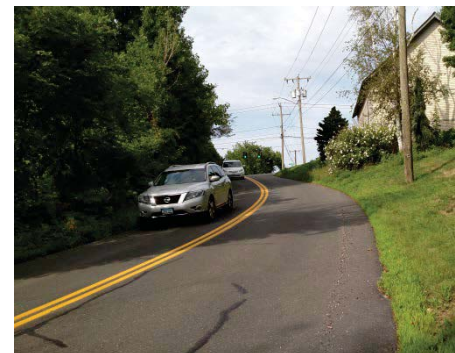
Figure 14. Narrow Curvy Road (Old Post Road)
