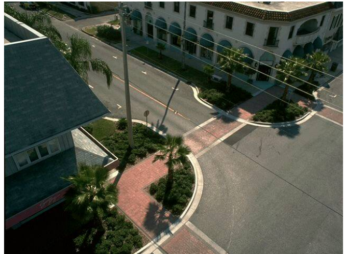
Figure 18. Typical Pedestrian Crossing Bump outs
