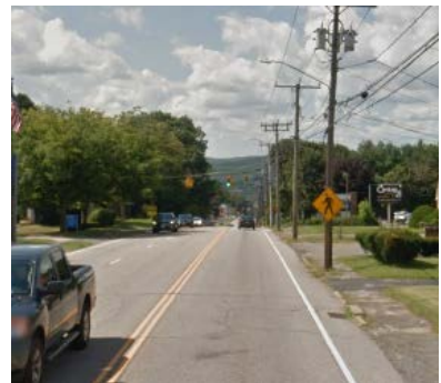
Figure 11. Pedestrian Crossing Sign not Near a Sidewalk
