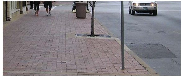
Figure 13. Example of Sidewalk Which Stands Out From Road
