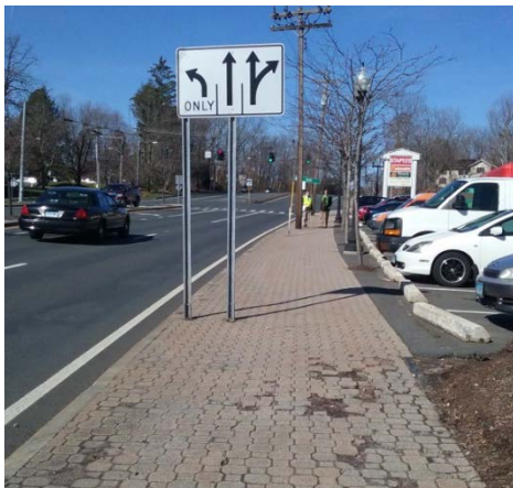
Figure 17. Repair Damaged Sidewalk Areas
