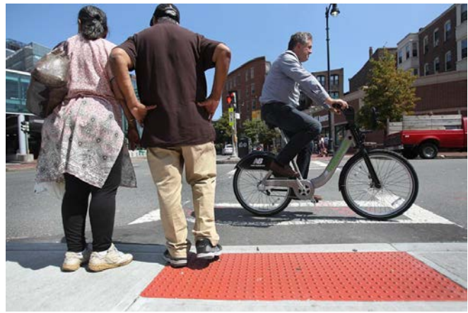
Figure 18. Example of Detectable Warning Strips
