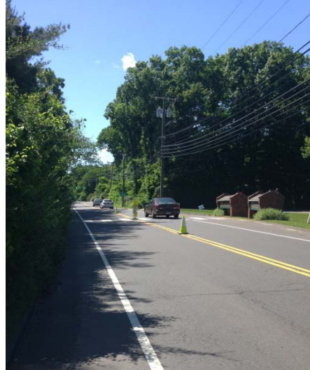
Figure 6. Pedestrian Crosswalk at Weston Center Plaza
