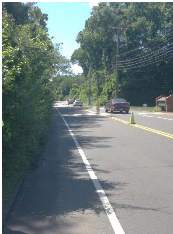
Figure 13. Trim Areas With Overgrown Vegetation
